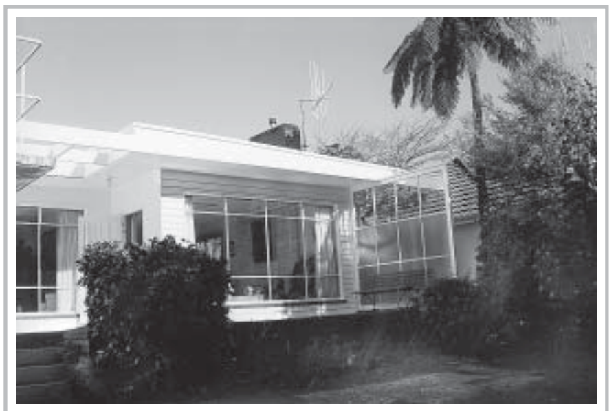
Large windows with metal frames and a terrace screen. McMillan house, Jickell St.
