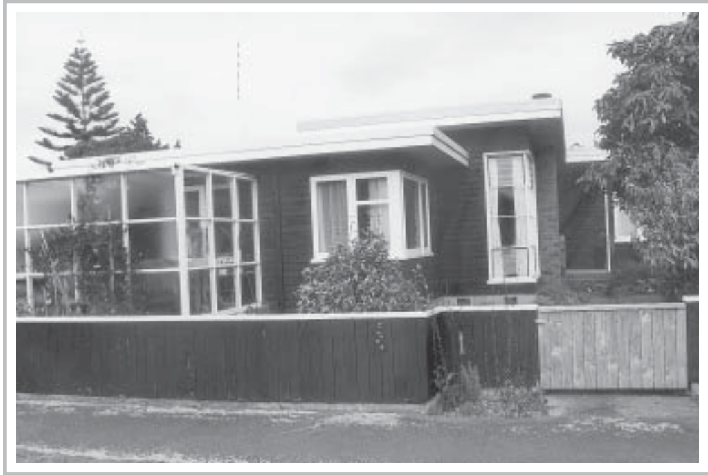
Weatherboards painted with creosote. Fife house, Hughes Ave.
