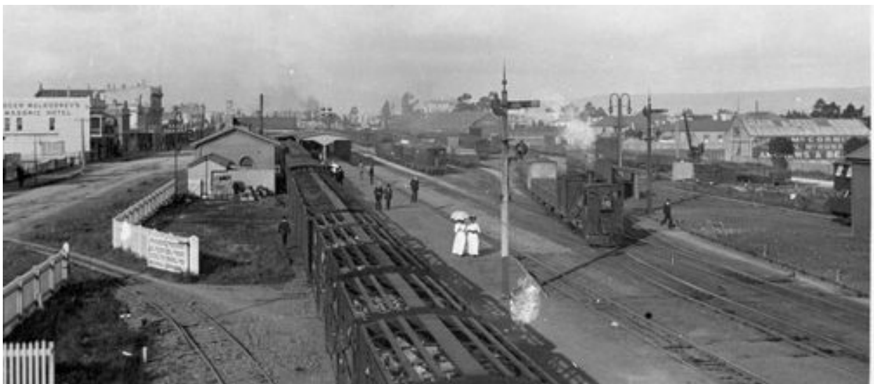
Palmerston North Railway Station and Yards c 1906.
